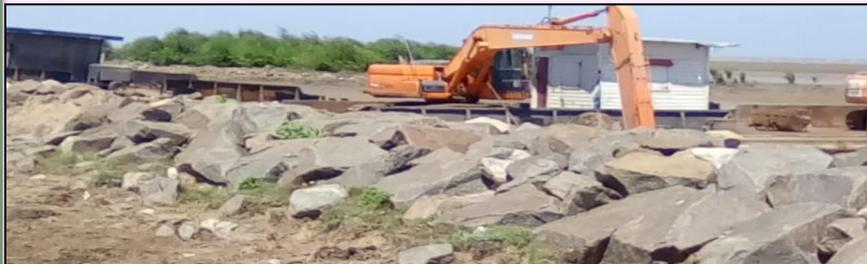
Photo: Reinforcement to protect a section of the coast from erosion by strong waves.
